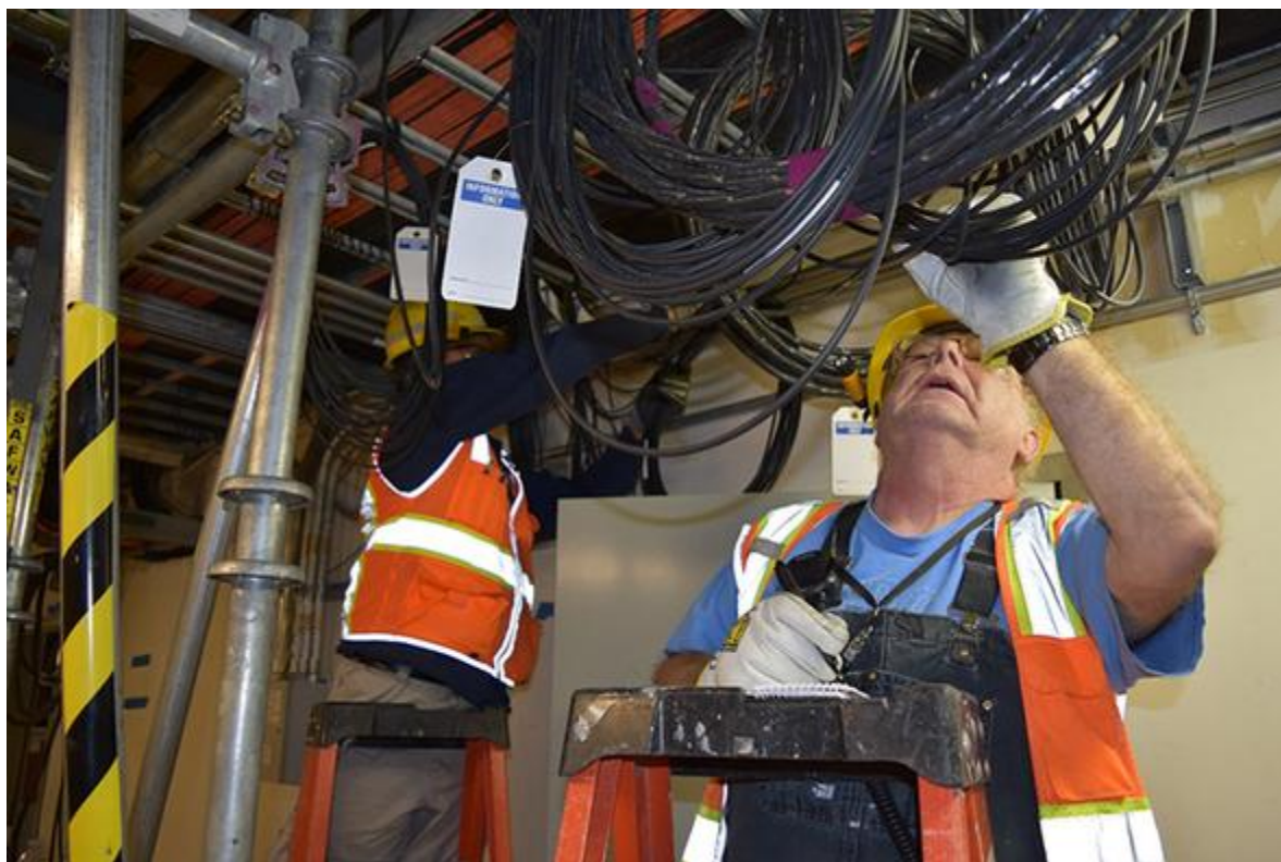
Hanford Waste Treatment and Immobilization Plant electricians install wiring inside the Low-Activity Waste facility.
